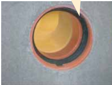
Water tight rubber seal
